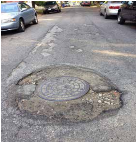
Figure 15. Periods of high temperatures soften and expand roadway materials, creating ruts, which are exacerbated by vehicles to create potholes. Photo: Nicholas Occhipinti
