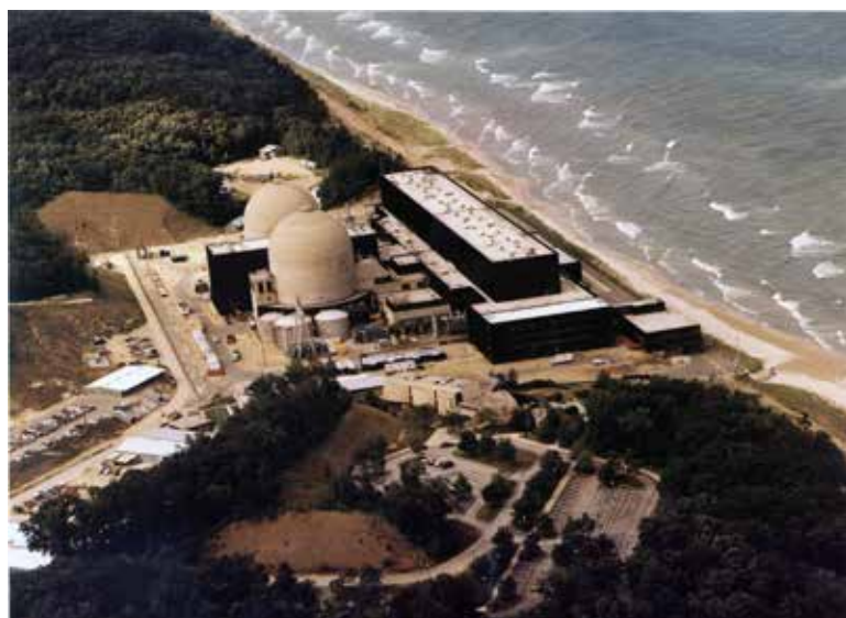
Figure 10. The D.C. Cook Nuclear Power Plant was shut down in July 2006 because of extreme heat.
