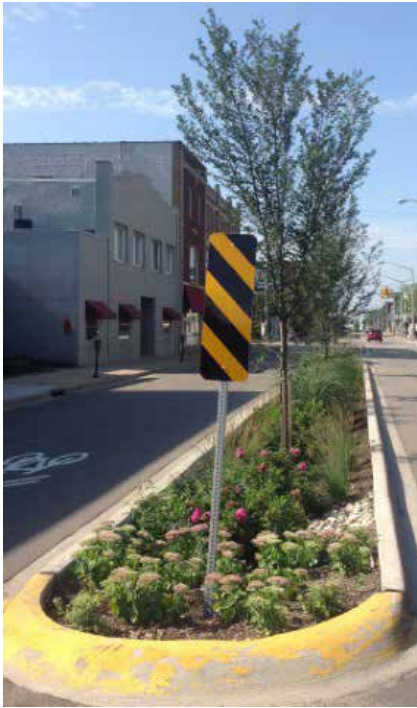
Figure 17. Plainfield Avenue bioswales are designed for stormwater infiltration, neighborhood beautification, and multimodal transportation safety.
