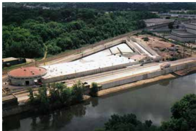
Figure 29. MARB prevents almost all direct discharge of untreated wastewater into the Grand River. MARB can store and partially treat 30 million gallons of wastewater per day.
